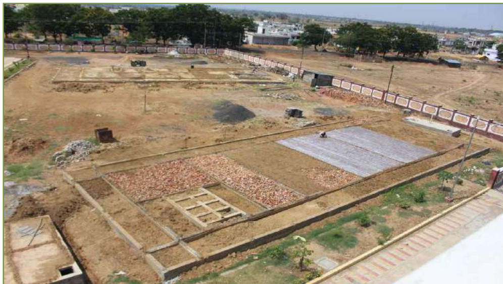
Present construction status of STR at Gondwana University, Gadchiroli
